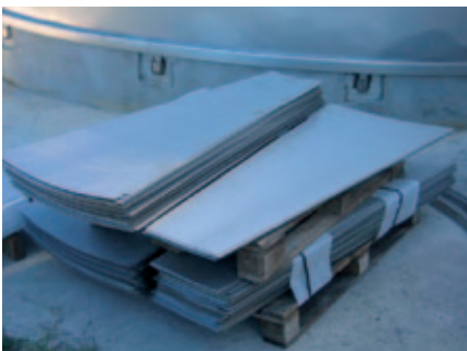
3) Segmented sections of the diaphragm, previously assembled: the segments are assembled at the workshop based on calculations performed on the technical drawing of the tank.
