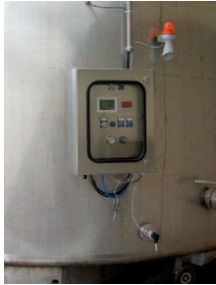
6) Installation of the electrical control panel from which it is possible to manage automatically the temperature, opening of the bypasses and the injection of technical gases (macro-oxygenation, \text{CO}_2 timer control for the pre-fermentative dynamic maceration).
