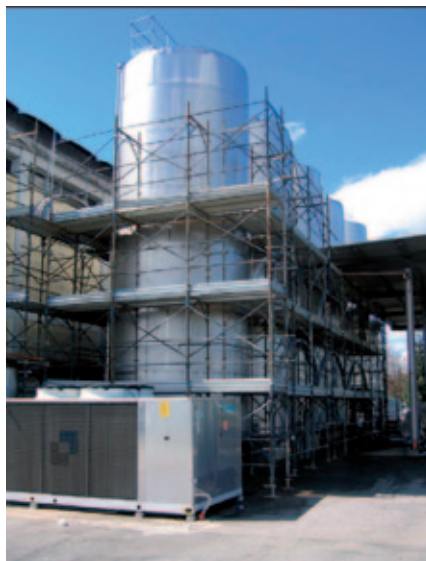
2) Scaffolding assembly: internal and external scaffoldings are necessary in order to weld safely the diaphragm, bypass valves and any external cooling pockets.
