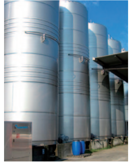
The process ends with a hydraulic test on the winemaker, in order to simulate all the stages that will take place at time of grape harvest.
