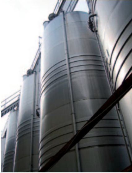
5) Welding of the cooling pocket on the plating: if necessary, the tank is thermal conditioned through the application of channels or mantle-shaped pockets, which are welded on the tank cylinder.
