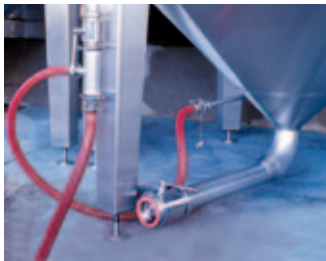
Conical bottom with «Sluice Point» device
